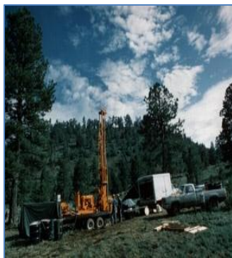
SCIENTISTS USED HYDRAULIC FRACTURING TO CREATE A HEAT EX-TRACTION LOOP IN THE HOT GRANITIC ROCK UNDER THE JEMEZ PLATEAU IN NEW MEXICO. (Photo with permission from the U.S. Department of Energy)
