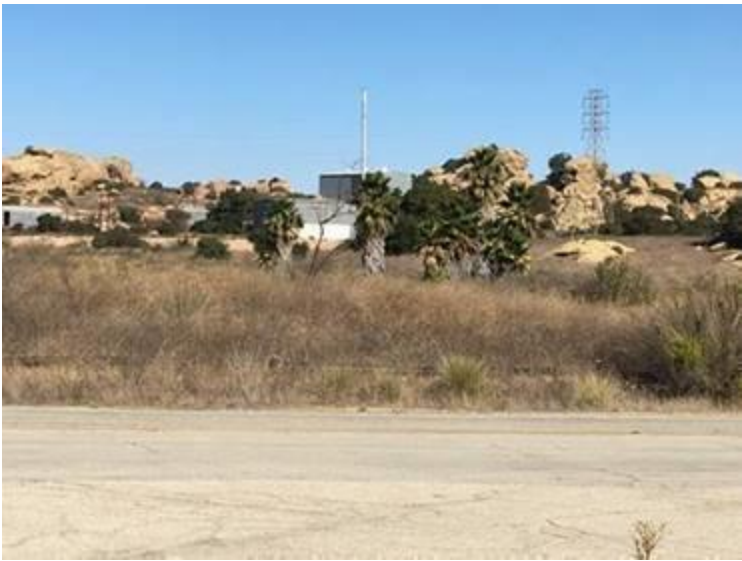
Powerlines, DOE buildings and roadways remain intact from Woolsey Fire
