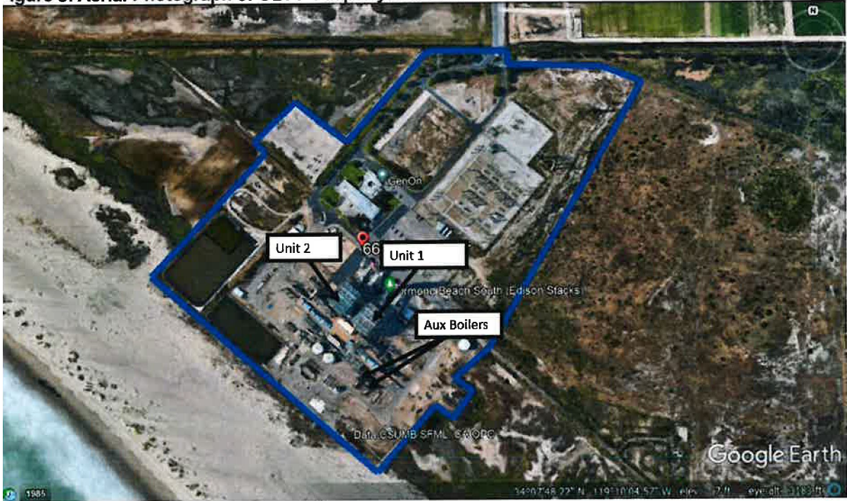
Figure 3: Aerial Photograph of OBPP Property and Fenceline
